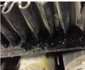
Sidewall belt repair
